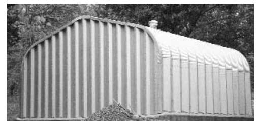
Solid endwall completed.
