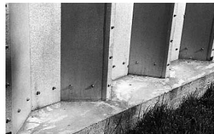
Trough or C-Channel after grouting.
