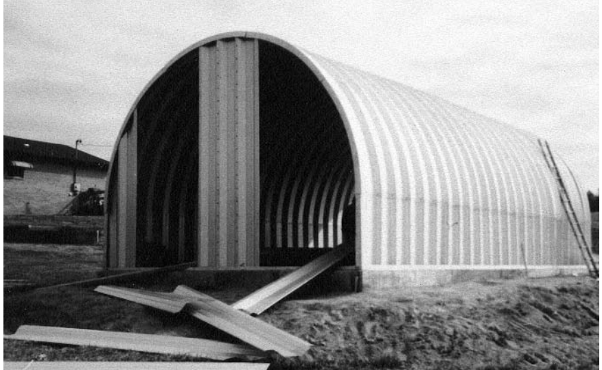
Solid endwall in progress.
