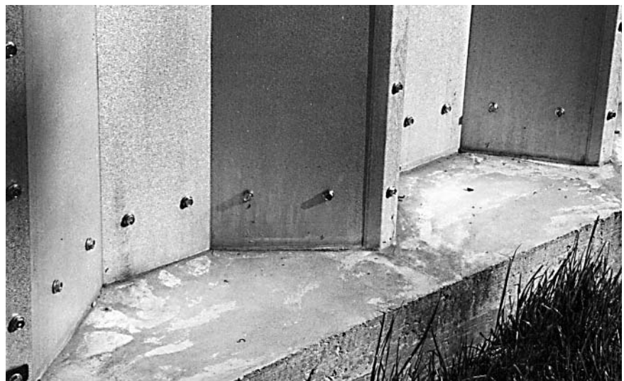
Grouting completed.
